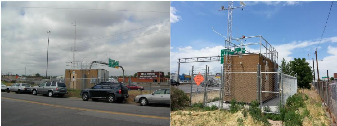
Figure 4. Pictures of Existing Denver Near-Road Monitoring Site (971 Yuma Street)
