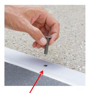
Although this type of ramp is meant to be portable, be sure it is secure so that the ramp does not slip out of position when someone is using it. Also, consider the weight limitations of the portable ramp.
