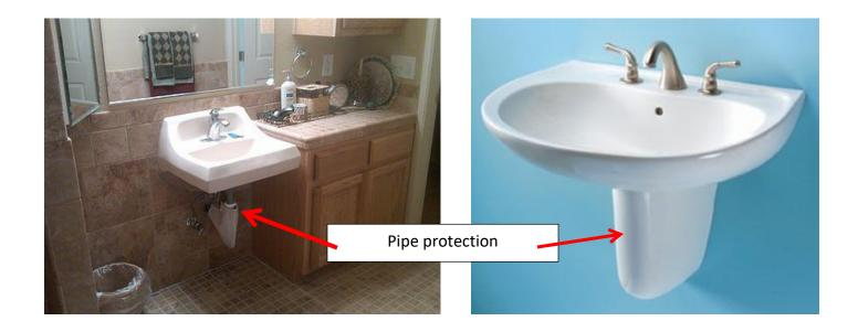
Pedestal Sinks come in a variety of styles and sizes. Consider the pedestal and how it can impede a wheelchair.
