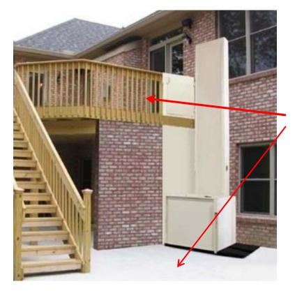
Be sure there is an accessible route to the lift and that there is enough room for someone in a wheelchair to access the lift from the top and bottom!
