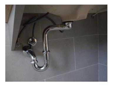
Create more space under the sink by using an off-set drain
