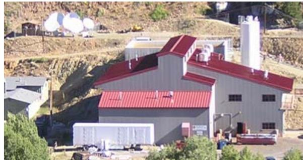
*Before and after images of the Argo Tunnel Water Treatment Facility in Idaho Springs. The most visible change will be a new thickener tank outside the existing building, below. Two existing clarifier tanks inside the facility will be repurposed as reaction tanks, which may actually increase plant capacity. The conversion project will reduce waste, boost efficiency and save money.*
