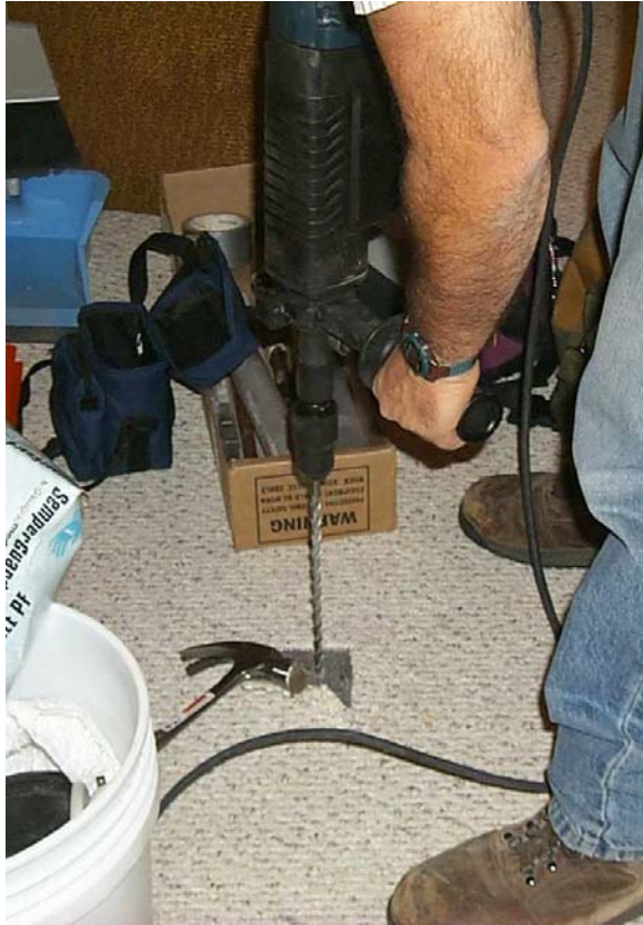
Figure 1. Drilling through a slab
