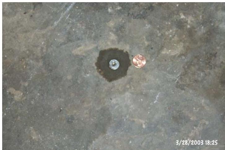
Figure 5. Completed vapor probe installation
