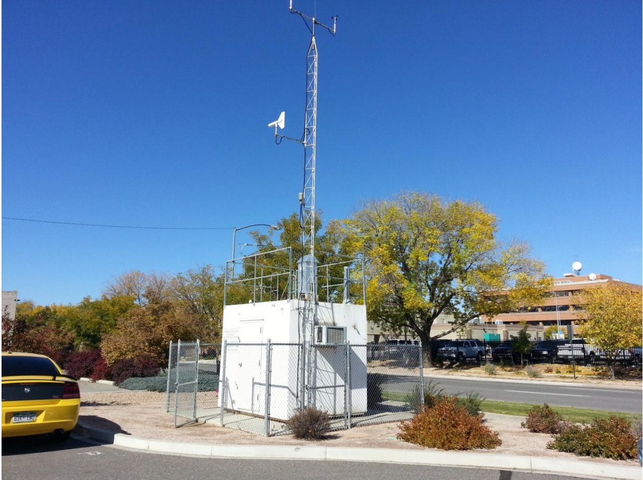
Site Photo: Shelter and inlets (looking NORTHWEST )
