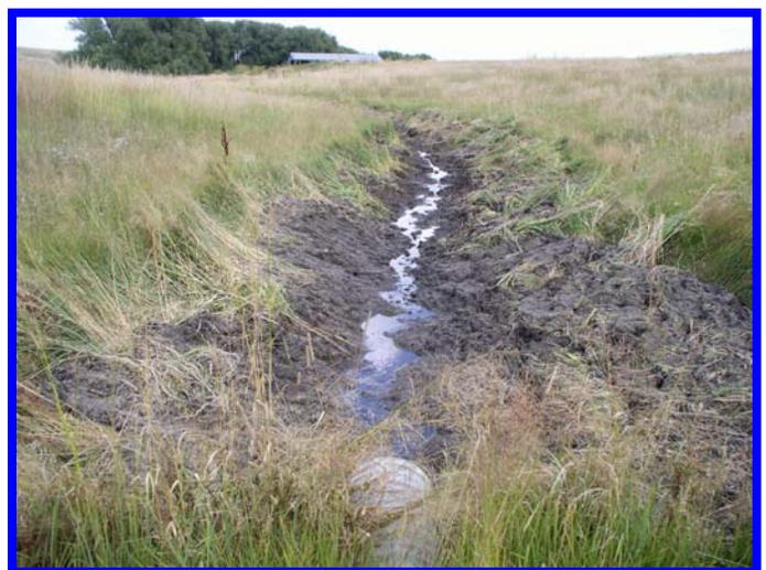
*Small earthen dams protect against potential floods that could cause millions of dollars of damage to residential and agricultural land in the Kiowa Creek watershed. On the left, the picture shows an outlet pipe from such a dam without a positive grade and that was half under water. On the right, the picture shows water draining freely away from the dam once the outlet channel has been cleaned out.*
